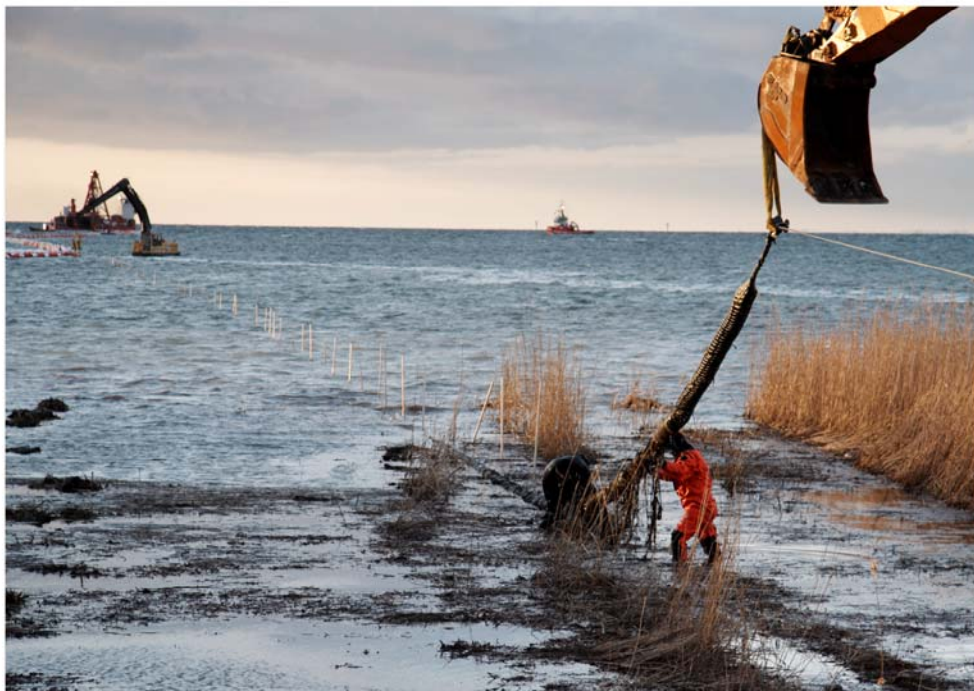
Lillgrund Wind Power Plant 2006-12-18 Submarine export cable installation. Pull-in at landfall.
