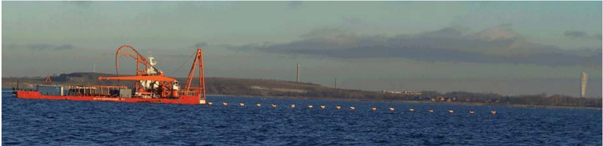
Figure 12. Inflated airbags took the cable towards shoreline.
