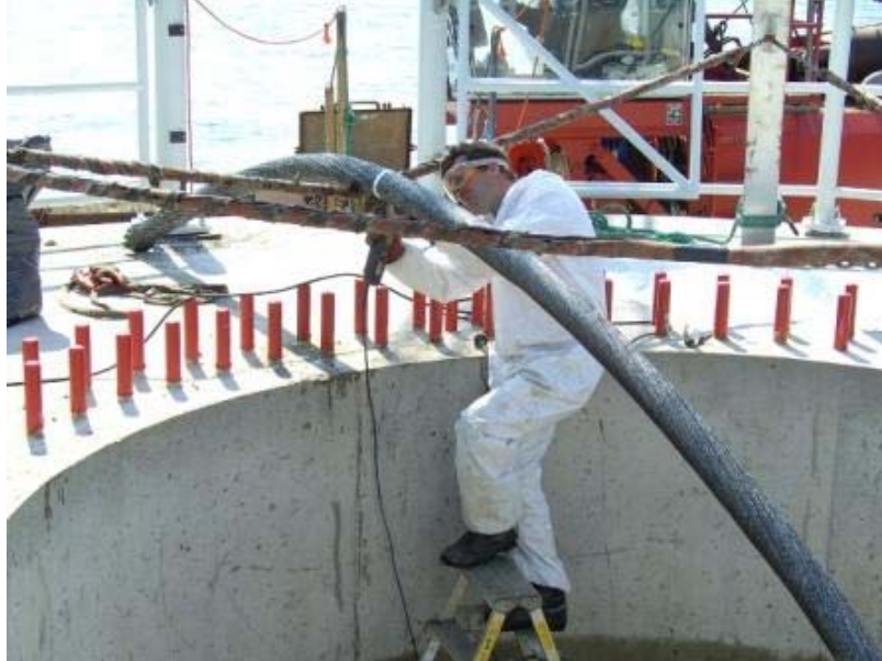
Figure 26. The cable armour was removed with help of an angle grinder
